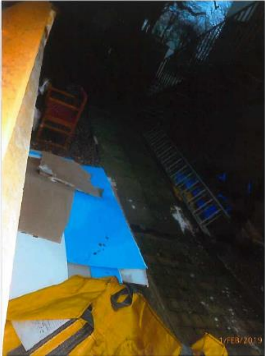
Physical damage and emergency exit
